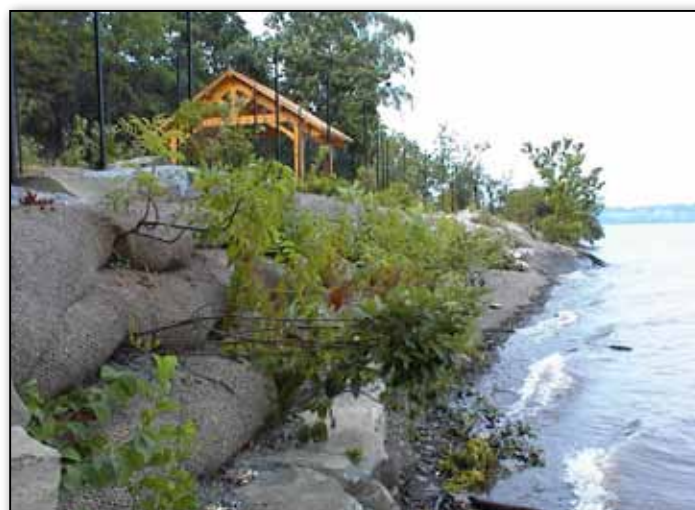
Installed vegetated shoreline stabilization treatment with native plant species, biodegradable soil bags, and a sloped shoreline.
