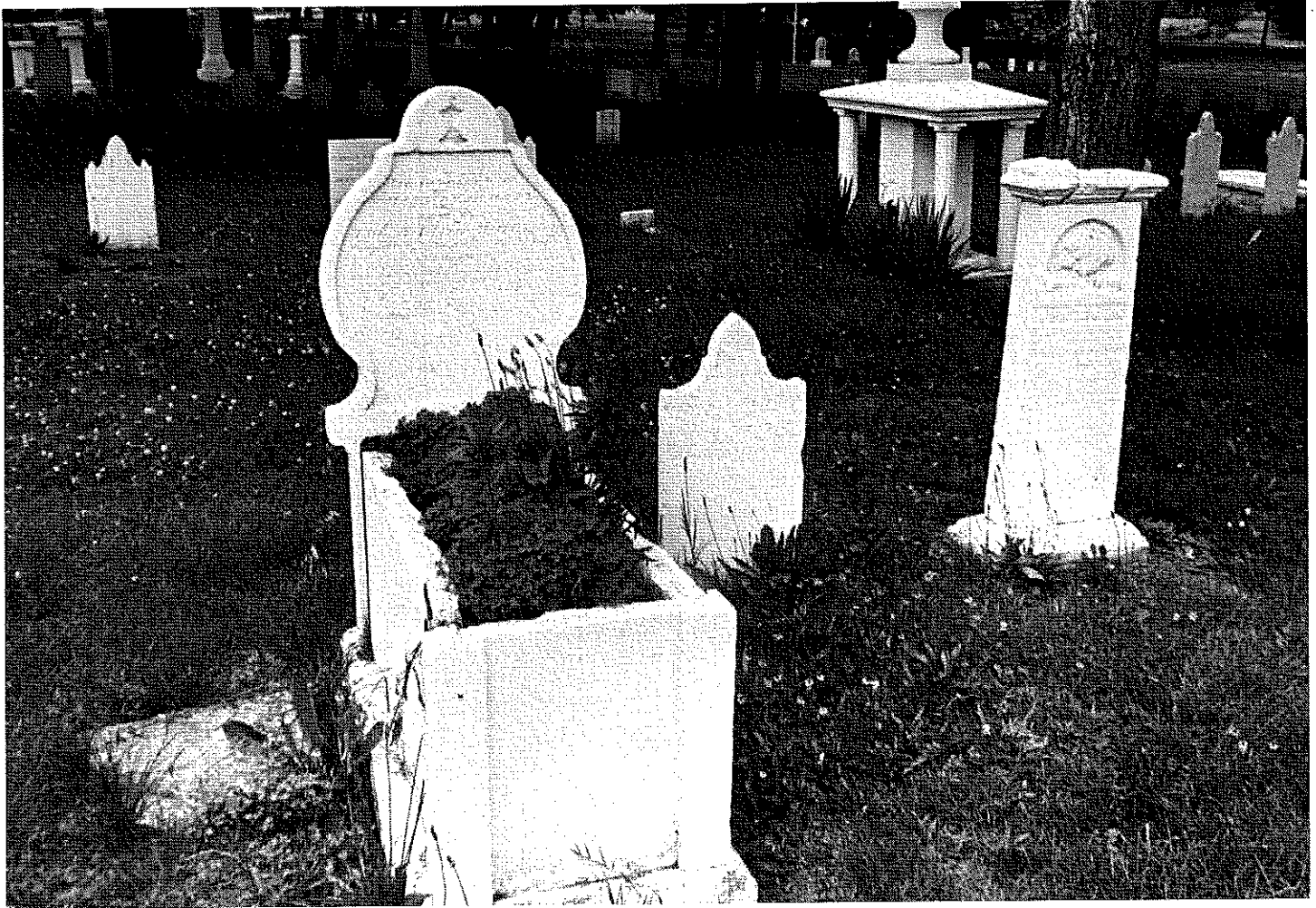
Pioneer Cemetery probably after a cleanup in the 1930s spearheaded by John B. Rodes. Although it appears that these stones have been cleaned, they were actually painted white. This is not a preservation method and is strongly discouraged. Photo courtesy of Special Collections Library, WKU.
