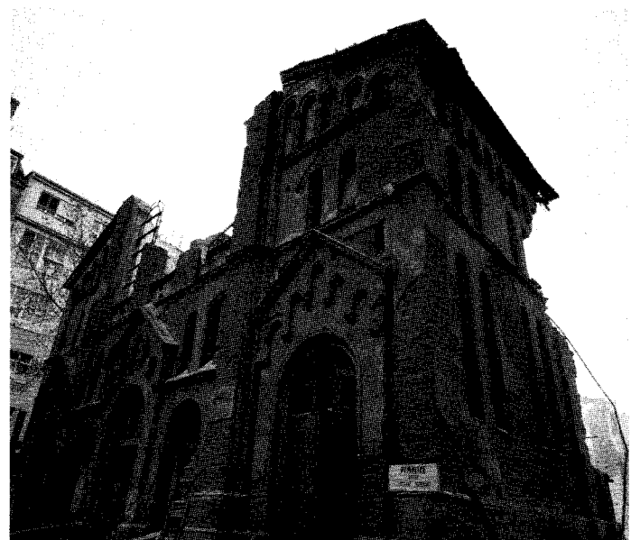
Demolition of synagogue. Brno (Czechoslovakia), 1986. (photo: E. Owen)
