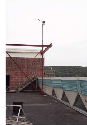
Photograph of Valders roof Anemometer
