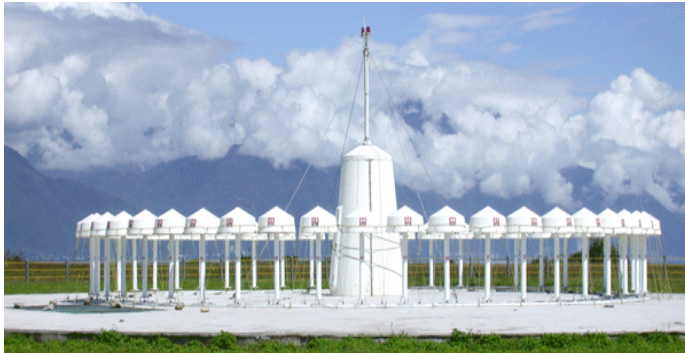
Figure-5.15 VOR-DME GND station left:[K4-6] right:[K5-1]
