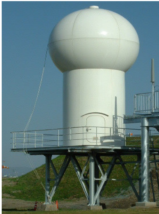
Figure-5.19 TACAN GND station [K4-7]
