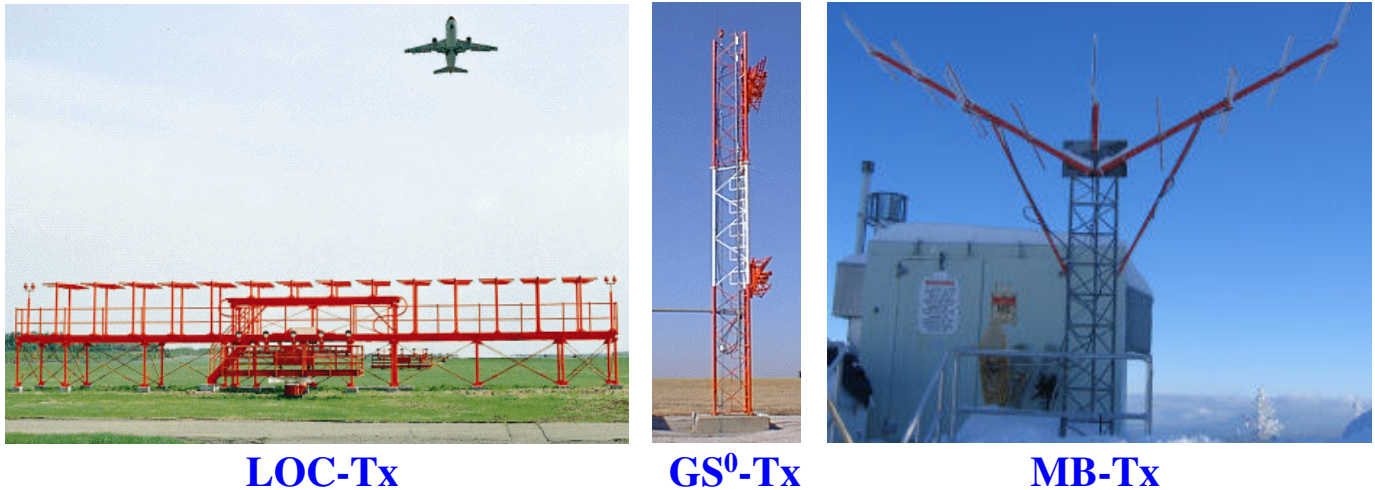
Figure-7.11 LOC, GS 0 , and MB-Txs [K5-5]
