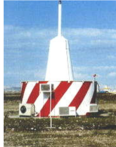
Figure-5.14 DME GND station left:[K3-17] right:[K4-5]
