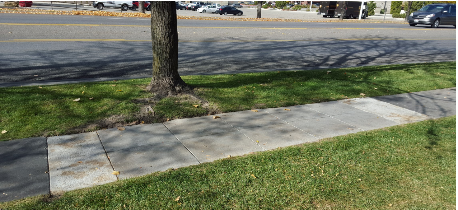
Another sidewalk installation site in Logan located at 1300 North 200 East. The close proximity of the Cache Valley Mall and Logan Pointe Apartments made this sidewalk a high priority for Logan City officials after the adjacent tree had buckled the old sidewalk in multiple places.
