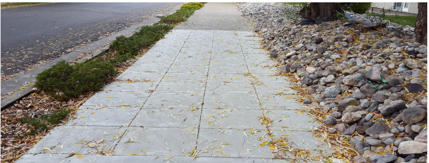
One sidewalk installation site in Logan located at 500 W Fairway Lane. Willow trees to the east were able to stay in place because the sidewalk tiles were used to replace the sidewalk that had been damaged by the tree roots.
