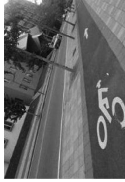
31. Cycle tracks are protected from adjacent travel lanes through curb separation, a buffer, or parked cars.
