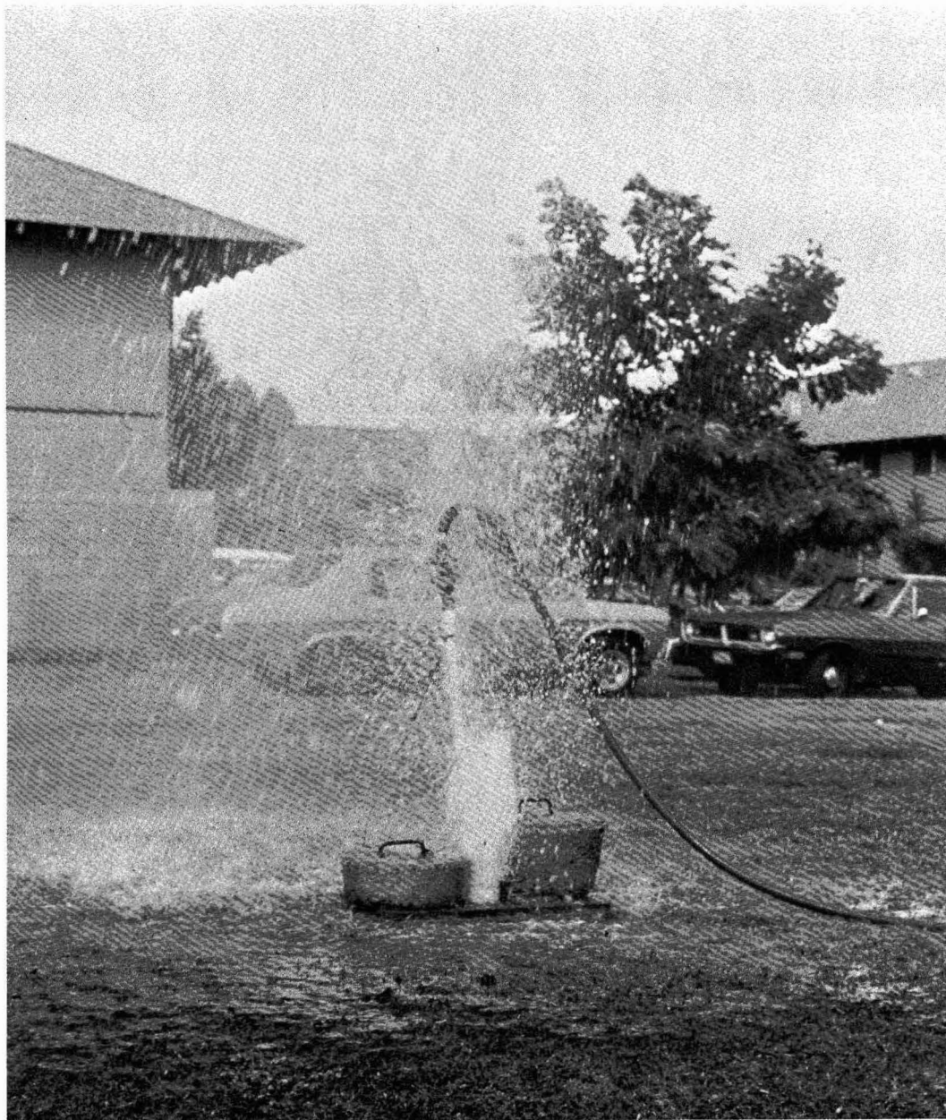
FIGURE 2. Compressed air used to unclog injection well, Ewa Beach, Oahu.
