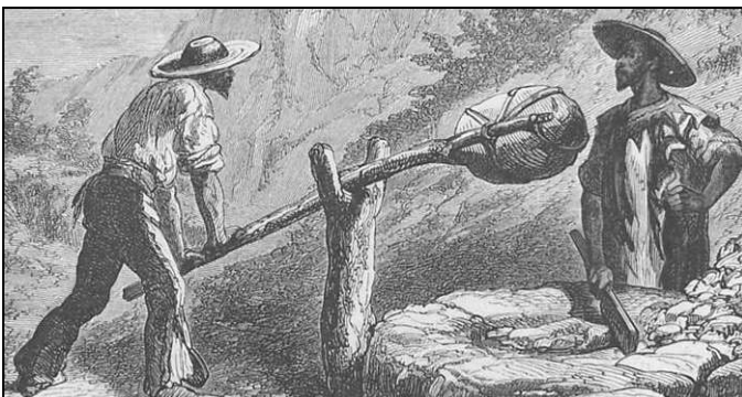
Figure 13. Crushing of ore during colonial period using a maray .
