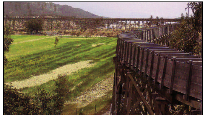
Figure 40. Transportation of tailings at El Teniente.
