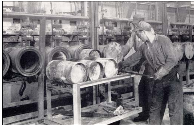
An operator collecting the magnesium from the condenser, 1940s
