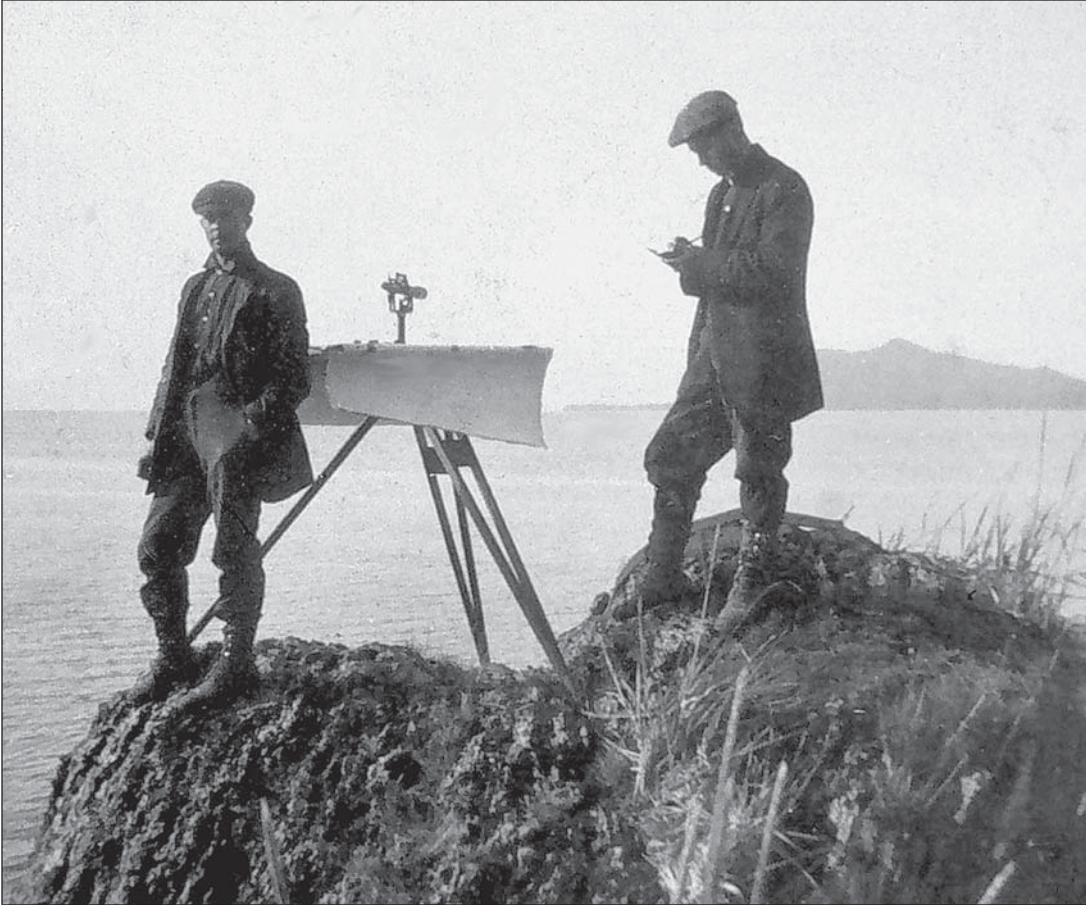
Coast survey teams chose prominent shoreline points for mapping stations. Plane table mapping, shown here at Prince William Sound in 1910, followed triangulation. Points were relocated using the surveyors' notebooks with descriptions of stations.
