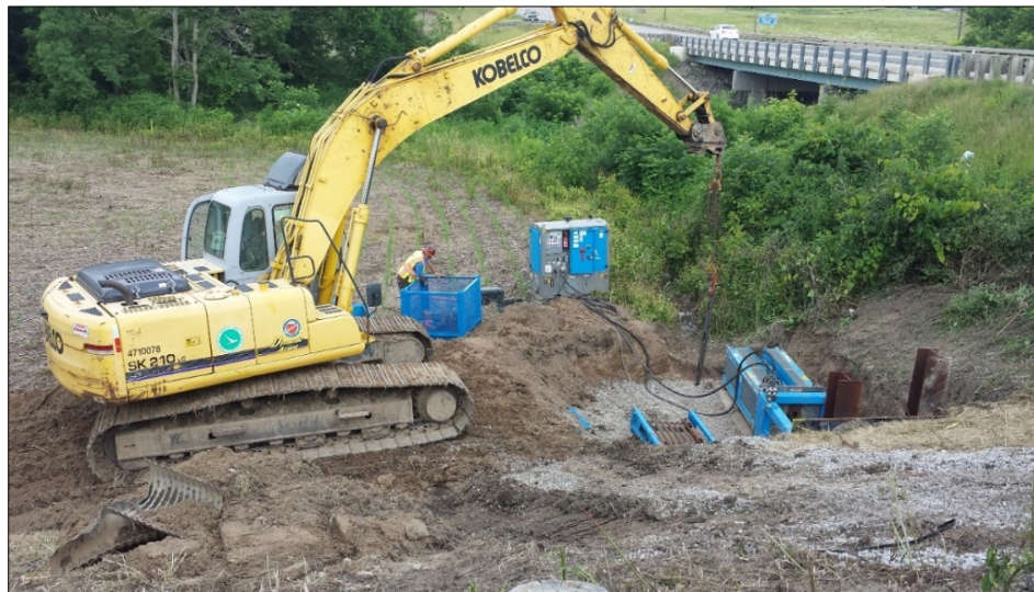
Figure 7a: System setup for static bursting
