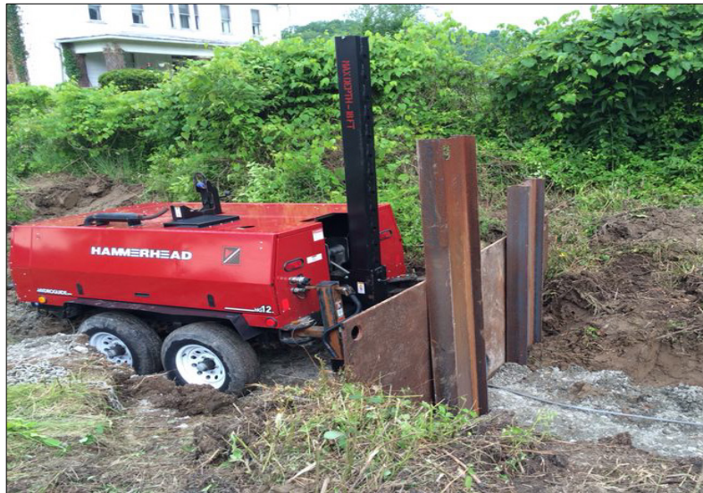
Figure 2: Winch Setup for pneumatic bursting
