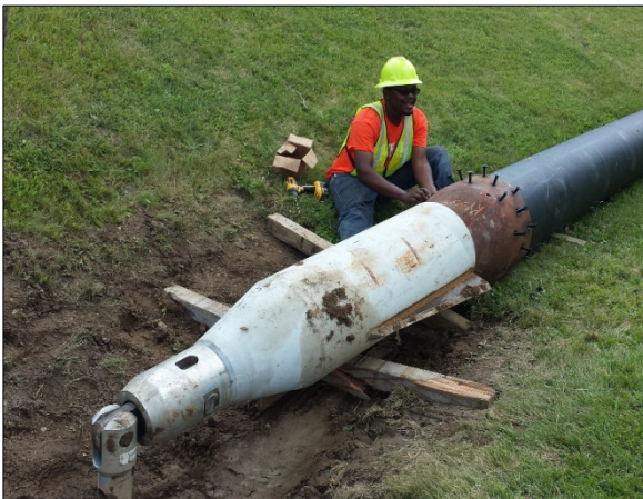
Figure 8: Bolting expander with bursting head on HDPE pipe
