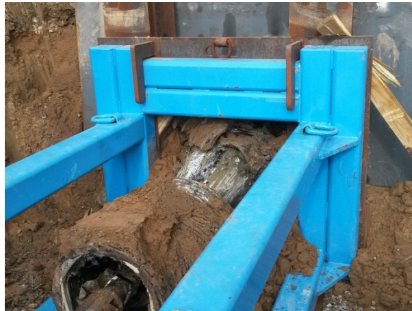
Figure 9: Folded CMP on bursting head
