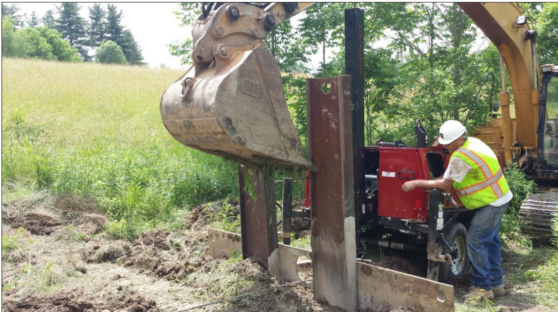
Figure 5: Setup with excavator supporting the I beams and steel plate
