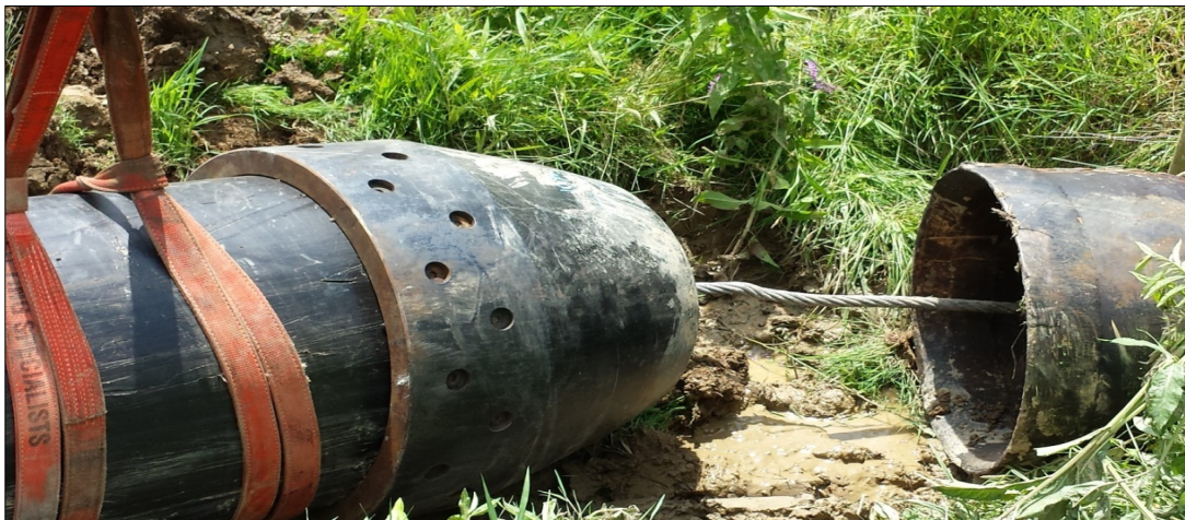
Figure 3: Front-end expander bolted to HDPE pipe with bursting tool inside the pipe
