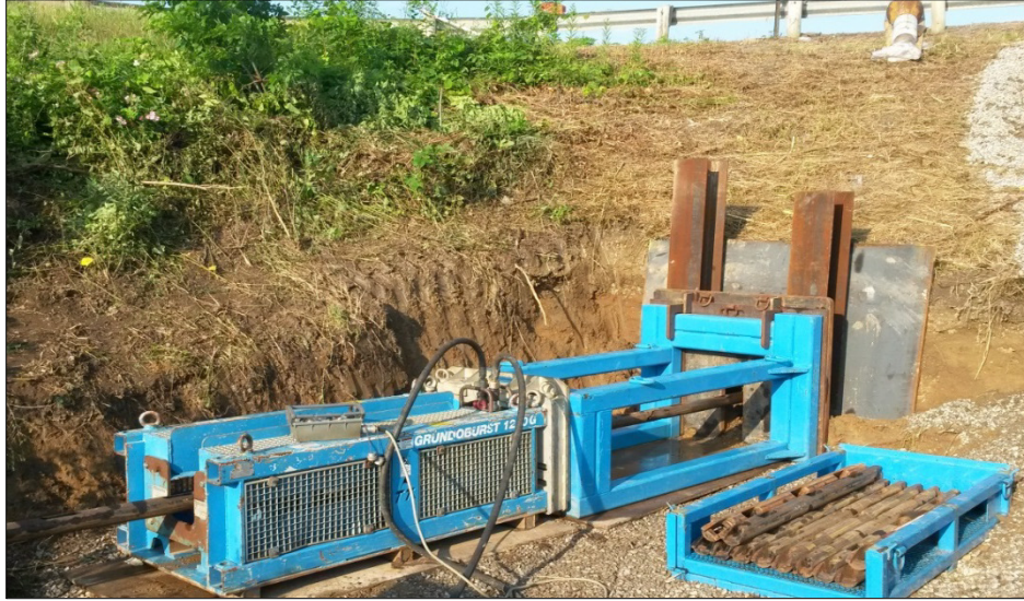
Figure 7b: System setup for static bursting
