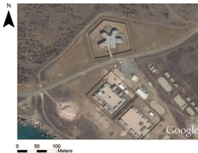
Figure 4 Satellite image of eastern edge of Camp Delta in November 2004, showing Camp Echo (two compounds of rectangular structures, bottom of image) and Camp Five (five-winged structure, top of image) (Google Earth, DigitalGlobe and Europa Technologies 2010).
