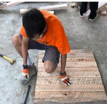
Student Fabricating Shutters and Door out of Formwork for Weather Station Building, Tanzania, Africa, Summer 2018
