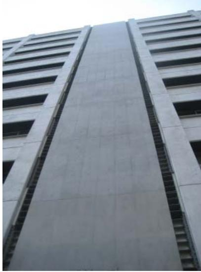
Figure 11. A central rocking wall as seen from the ground
