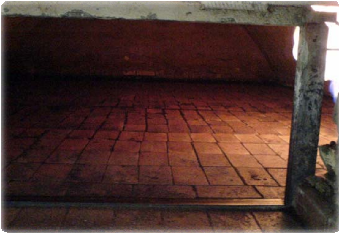
Figure 3. Interior of a Barbari oven, which is covered with Russian bricks.
