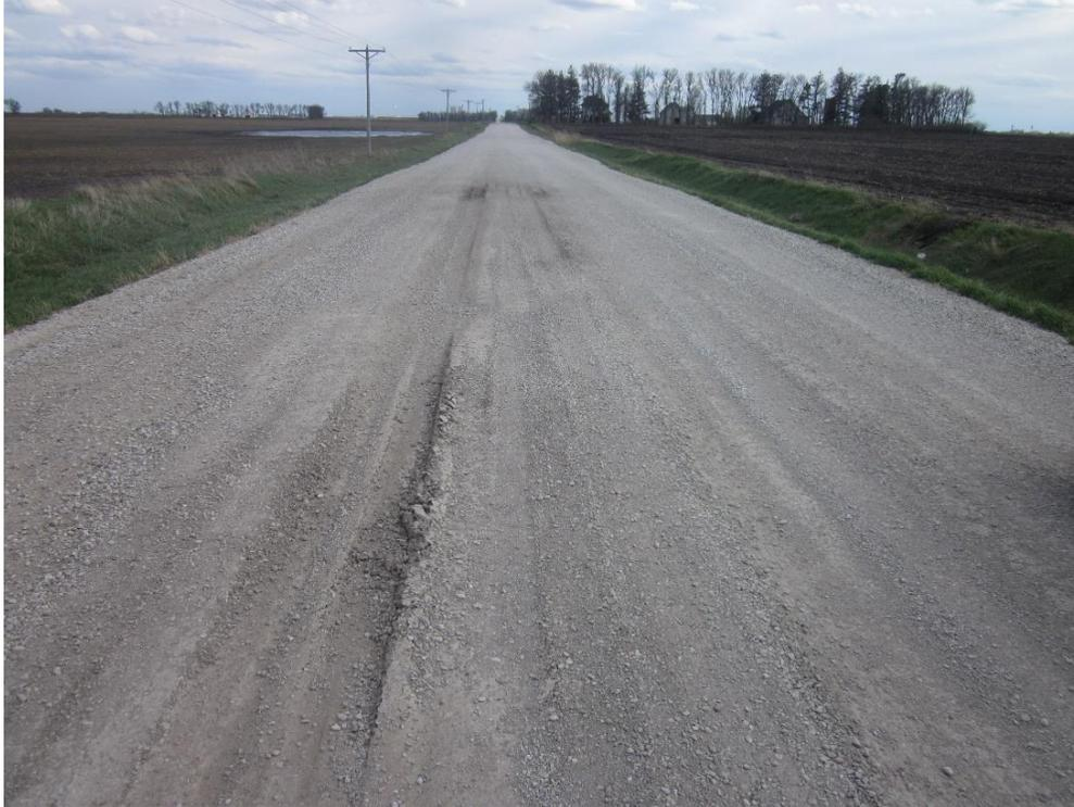
**Figure 102. Surface condition of geocomposite drain Section 18 showing rutting (April 21, 2015)**
