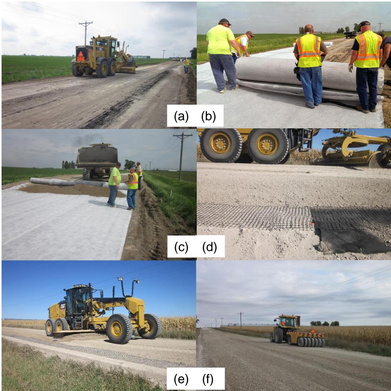
**Figure 42. Construction procedures and equipment for geosynthetically stabilized sections: (a) removal of existing surface, (b) geocomposite in Section 18, (c) replacement of surface course by earth mover for geocomposite Section 18, (d) BX geogrid in Section 19B on left with added non-woven geotextile in Section 19A on right, (e) replacement of surface course by motor grader for Sections 19A and 19B, and (f) compaction by rubber-tire compactor**
