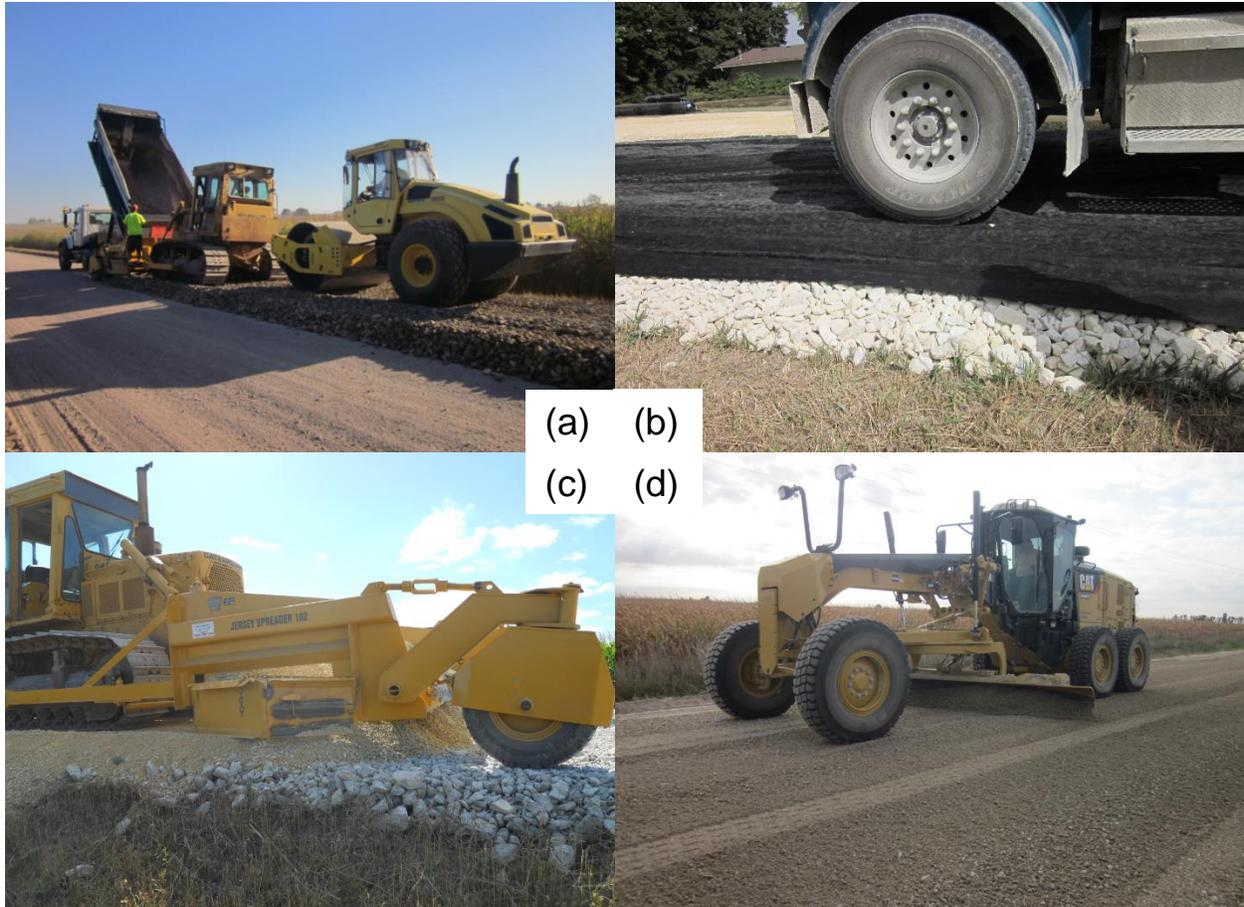
**Figure 37. Construction procedures and equipment for Sections 1-8 with macadam base courses: (a) placing macadam with Jersey spreader, (b) non-woven geotextile interlayer, (c) spreading choke stone with Jersey spreader, and (d) shaping with motor grader**
