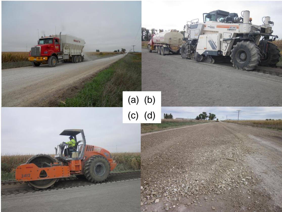
**Figure 40. Construction procedures and equipment for chemically stabilized Sections 15, 16, and 17: (a) powder truck for spreading bentonite, fly ash, and cement, (b) full depth reclaimer connected to water truck milling chemical stabilizers to the specified depth and water content, (c) vibratory pad-foot roller following the full depth reclaimer, and (d) 1 in.-thick road-stone wearing surface**
