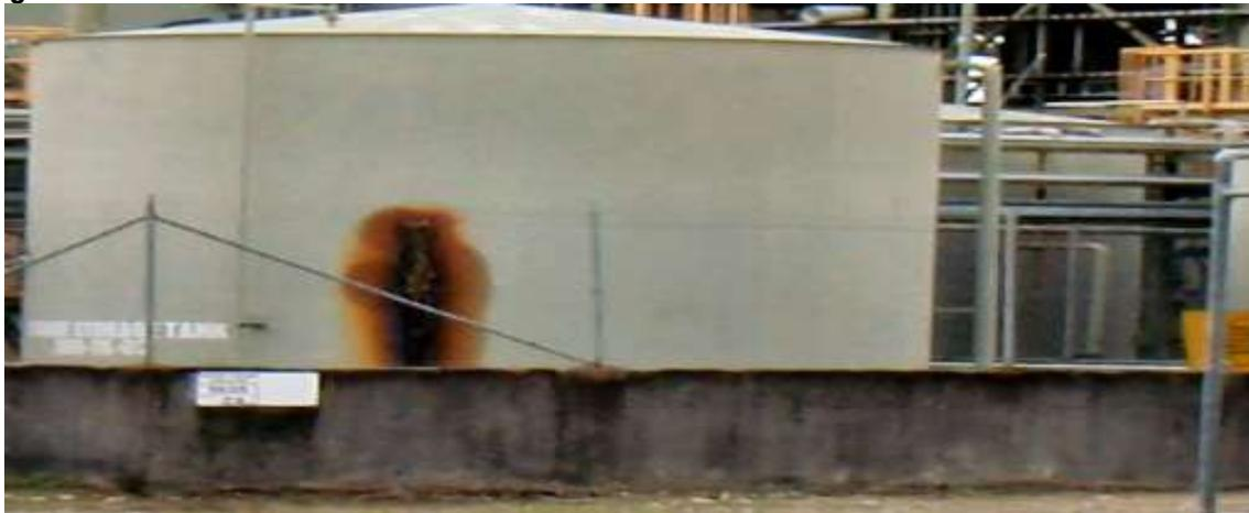
Fig 12: Cyanide leakage at the mining site
