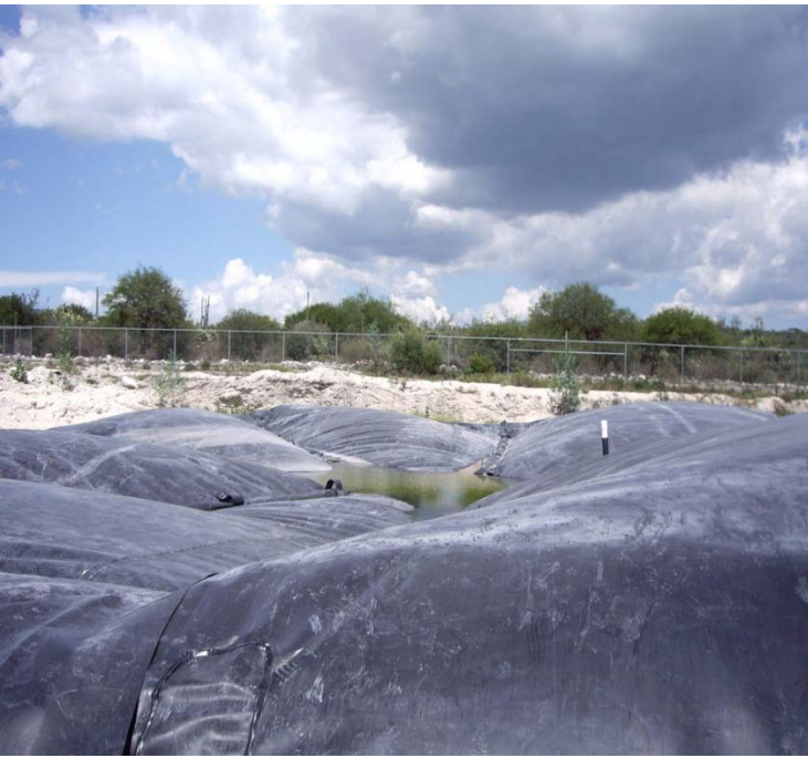
Normal positive pressure digester
