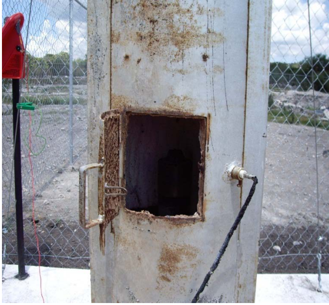
Flare not lit because backup pilot light cable burnt; 3 of the 6 digesters that the author visited did not have flares lit
