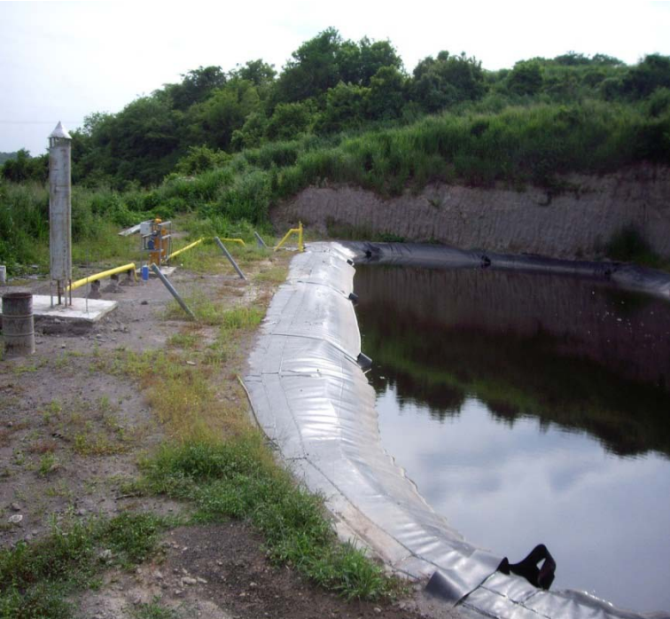
Positive pressure digester with water on top and no pump to remove it; consequently has low temps and producing no gas
