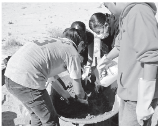
Image 1. Students mix concrete for the bench foundations.
