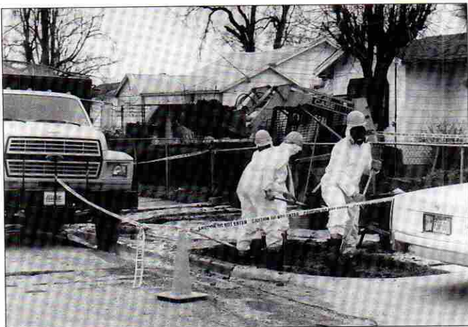
In a West Dallas, Texas, neighborhood, cleanup crews remove soil contaminated with lead from two nearby smelters.
