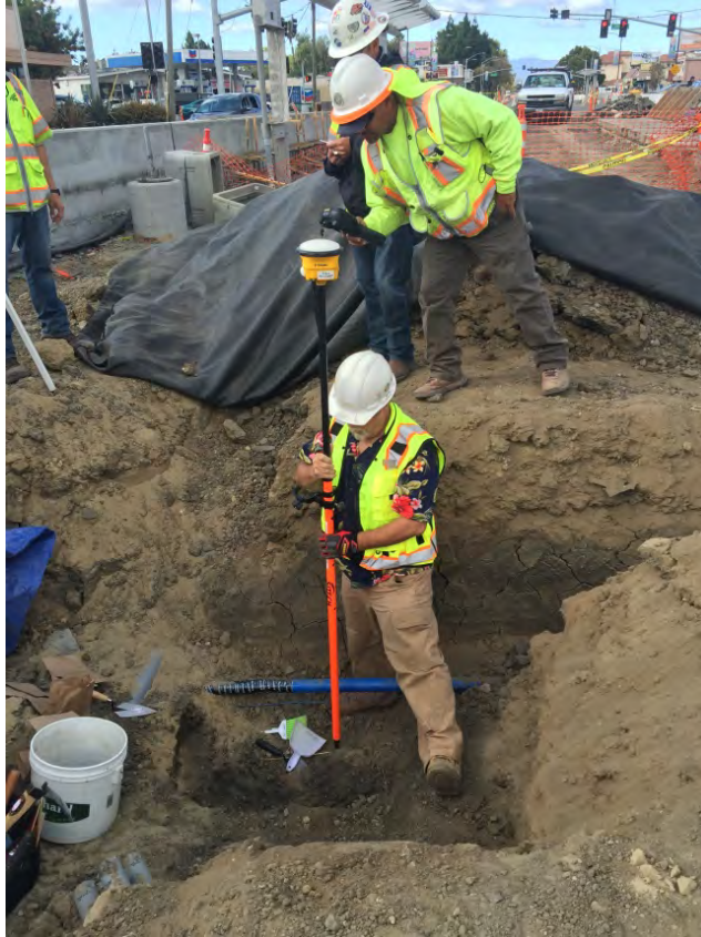
Figure 1-3: VTA Survey Crew Taking GPS Measurements
