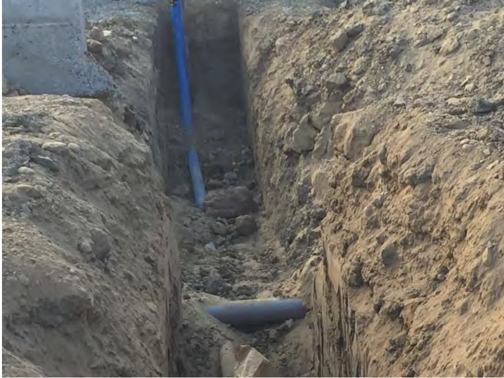
Figure 1-1: Fire Hydrant Trench
