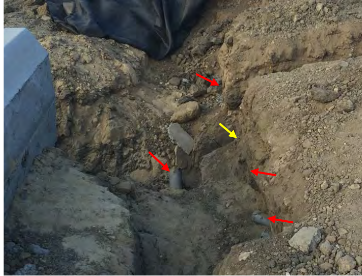
Figure 2-13: Trenching Activities around the Burial (red arrows indicate pipe locations; yellow arrow indicates Burial locus)
