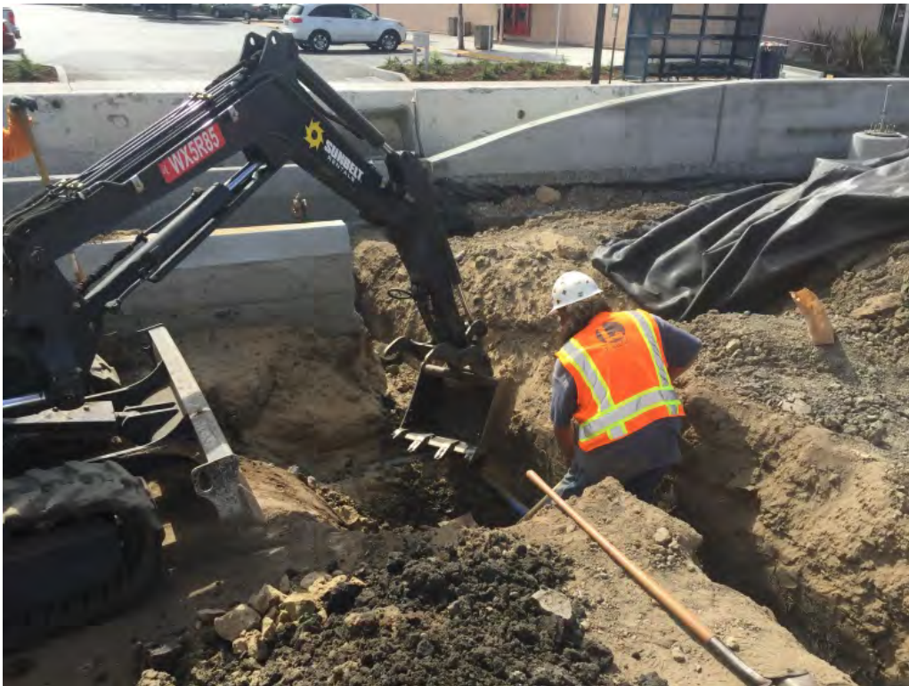
Figure 1-2: Small Backhoe Removing Overburden above the Burial
