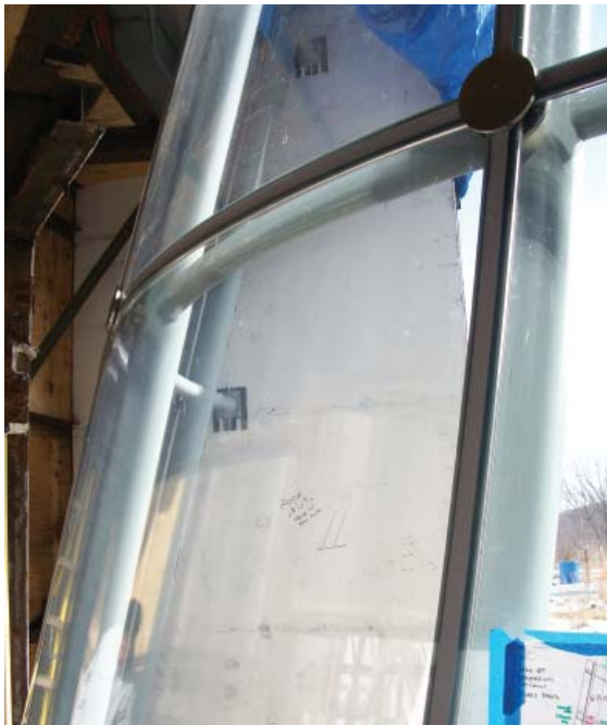
Figure 29: Patch fittings at the corner of glass units (left); Terrarium after construction (right). Photo credit Steve Hall © Hedrich Blessing Photographers.
